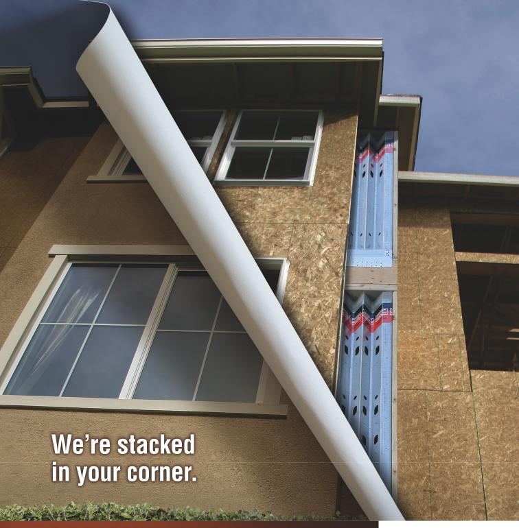
If you're planning to stack prefabricated shearwalls, make sure they're Steel Strong-Wall® shearwalls. The Simpson Strong-Tie two-story solution is not only code listed, but can be installed right at the corner to save wall space. And since our engineered shearwalls are available in widths as narrow as 15 inches for stacked applications, you can build multistory homes with larger windows, doors and open spaces without sacrificing strength and required load values.
